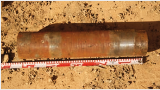
Image 18 Main pipe Qaraqosh, November 2016
